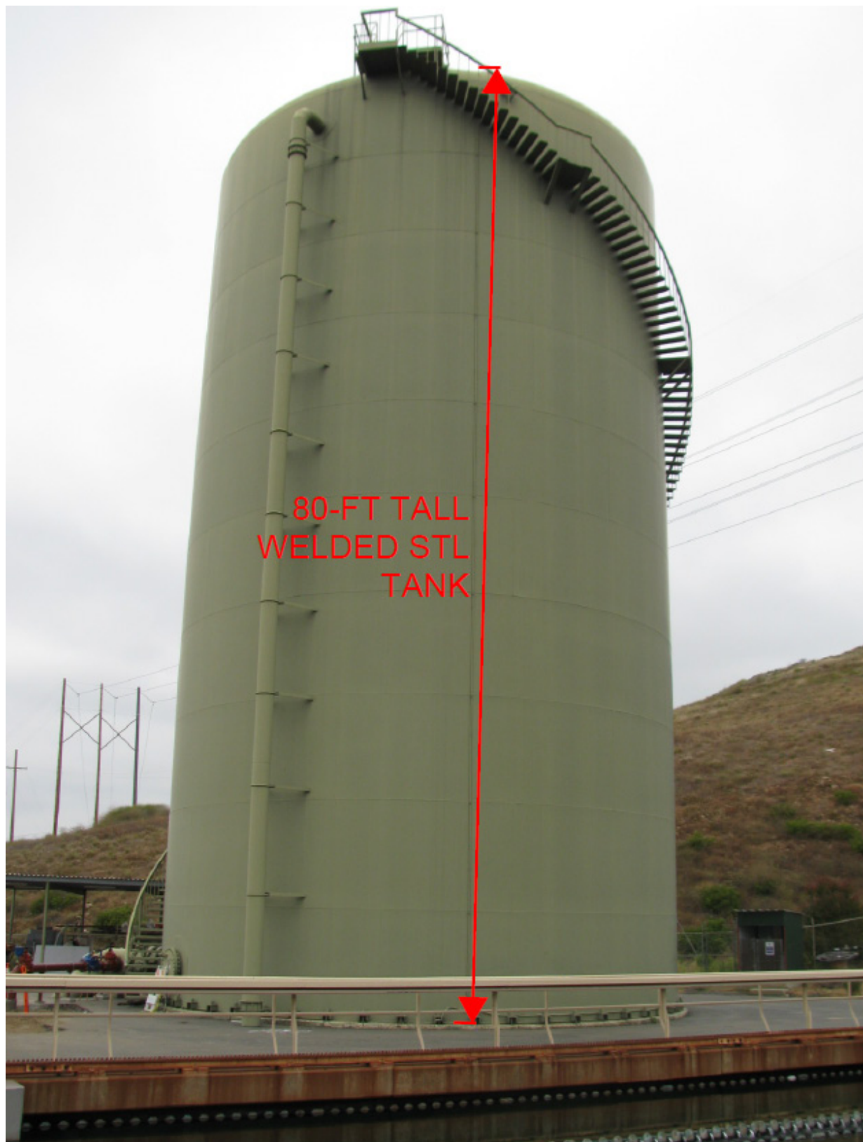
Figure H.1 The Backwash Water Tank is an 80-ft tall welded steel tank founded on a shallow concrete ringwall footing.
