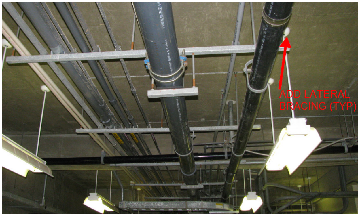
Figure H.9 Conduit and pipe hung from the ceiling of the Operations Bldg Basement lacks lateral bracing against seismic loads.
