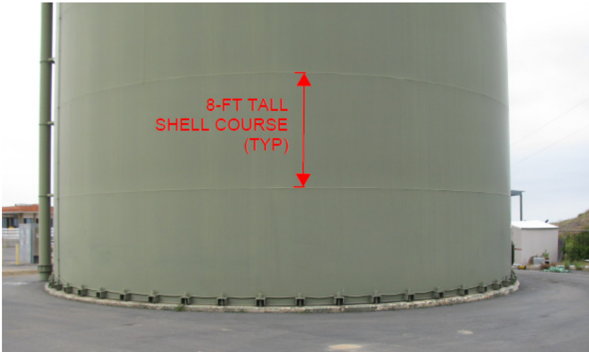
Figure H.2 The Backwash Water Tank is constructed with 8-ft tall steel shell courses.
