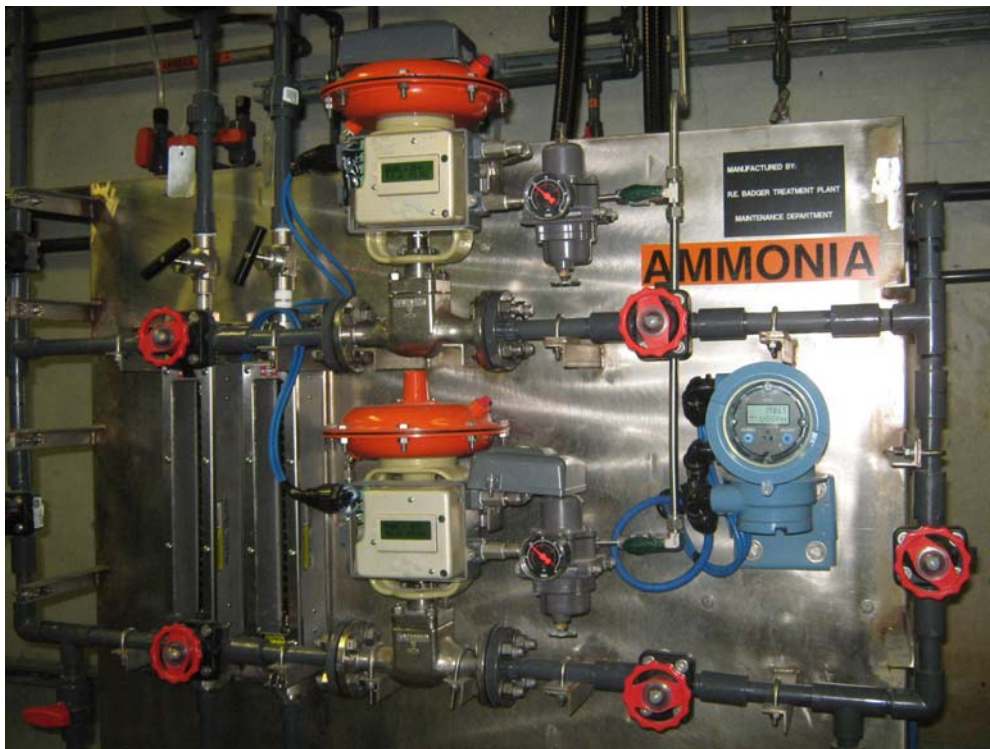
Figure 7.1 Ammonia Chemical Dosing Panel Designed and Manufactured by WFP Staff
