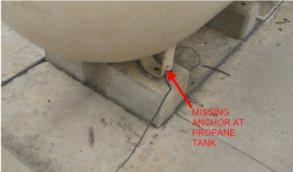
Figure H.5 The small propane tank at the chemical storage area is missing an anchor bolt.
