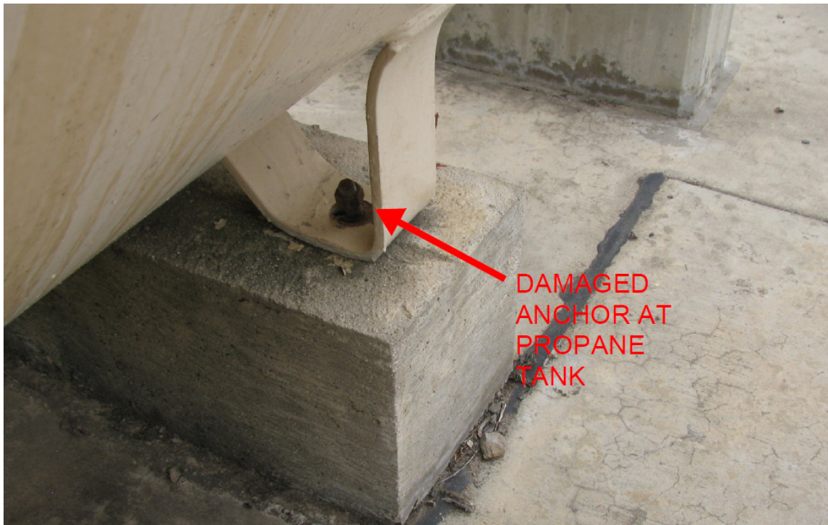
Figure H.4 The small propane tank at the chemical storage area has a damaged anchor bolt that requires replacement.
