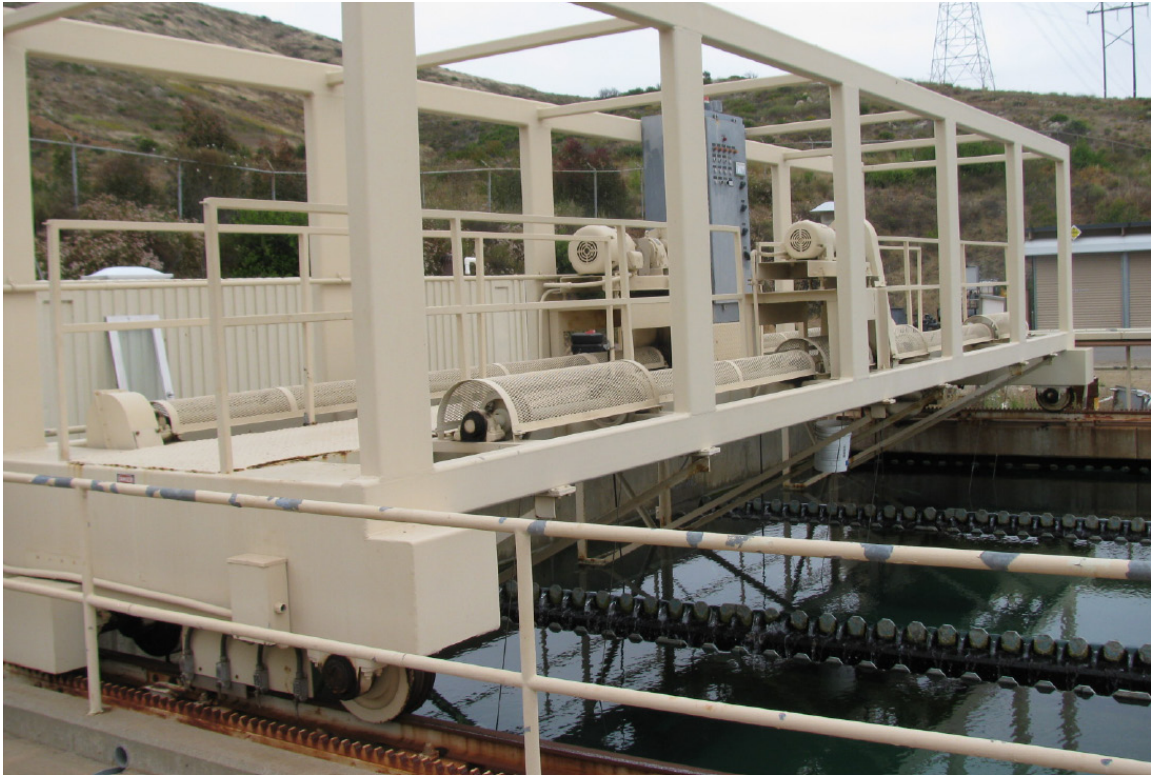
Figure H.6 The sludge collector mechanism rolls on a steel rail system.
